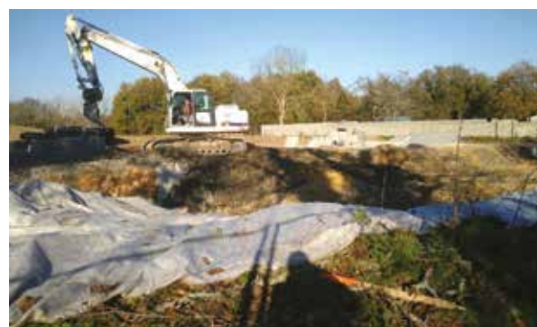
Construction caserne PSPG
